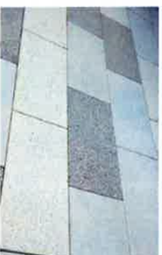
Granite Unit Paving
